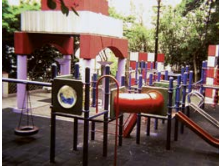
A Hard surface This attractive play area for children has a serious flaw: a concrete surface. The children may stay cleaner but are much more likely to sustain injuries with falls.
